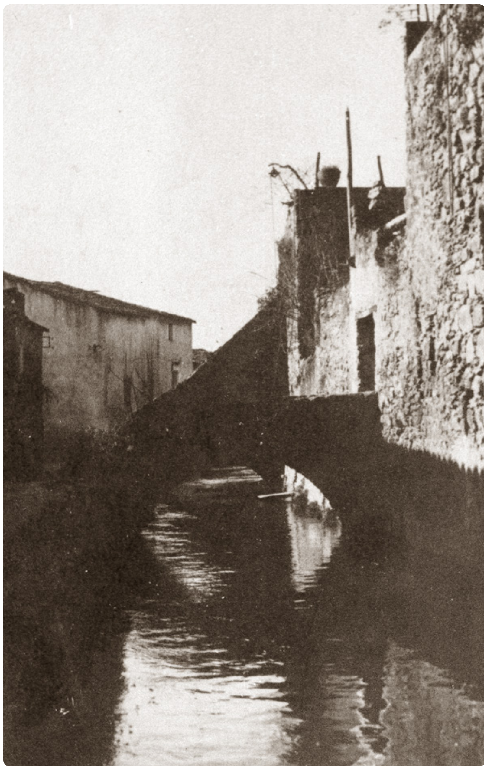
The mill leat following the curtain wall with one of the characteristic bridges to access the houses. Photograph by: Valenti Fagnoli. Source: Municipal Archive of Verges. Verges' Council collection.
