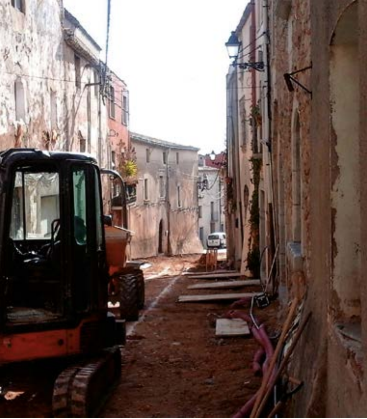
Obres al Carrer Major, 2017
